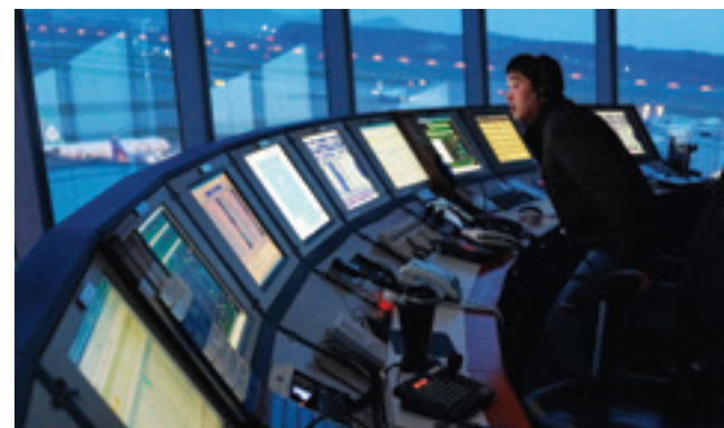
Air Traffic Control System
