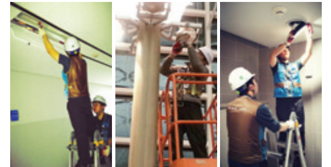
Replacing Lights with High-efficiency LED Lighting
